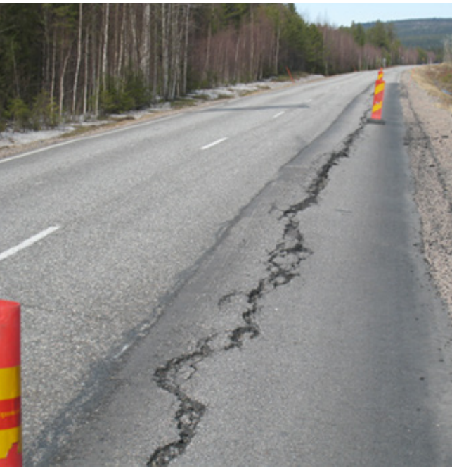
Differential frost heave between an old and a widened road section on road 934, Finland. (photo: Timo Saarenketo)
